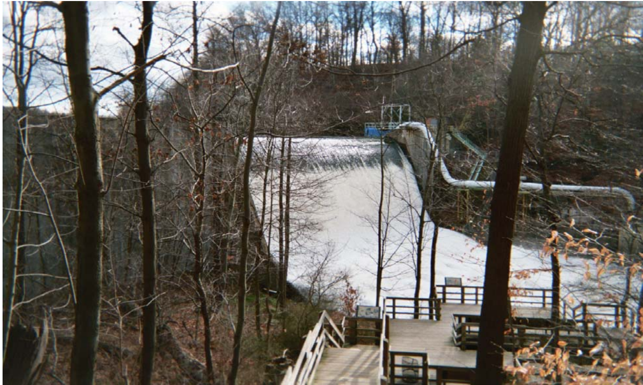
Photo 6: Dam viewed from north side. The wooden structure in the foreground is viewing platform in the park. The large white pipe is part of the experimental turbine that will be removed. December 4, 2004.
