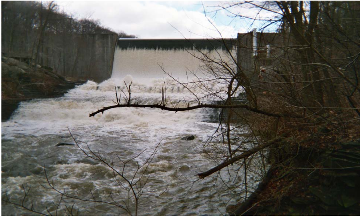
Photo 8: View of dam looking east. December 4, 2004.
